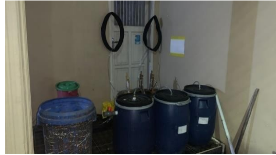
Gambar 7. Set Up Digester
